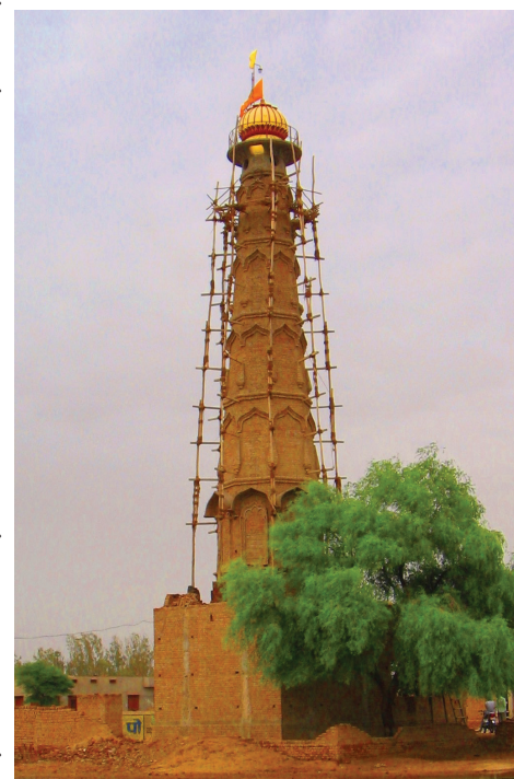
Figure 9: A tower temple under construction with baked bricks near Anupgarh. Photo: Author, February 2008
