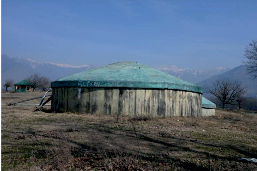
Figure 4: View of the water tank constructed on top of the archaeological mound at Gufkral (Image credit: Author)
