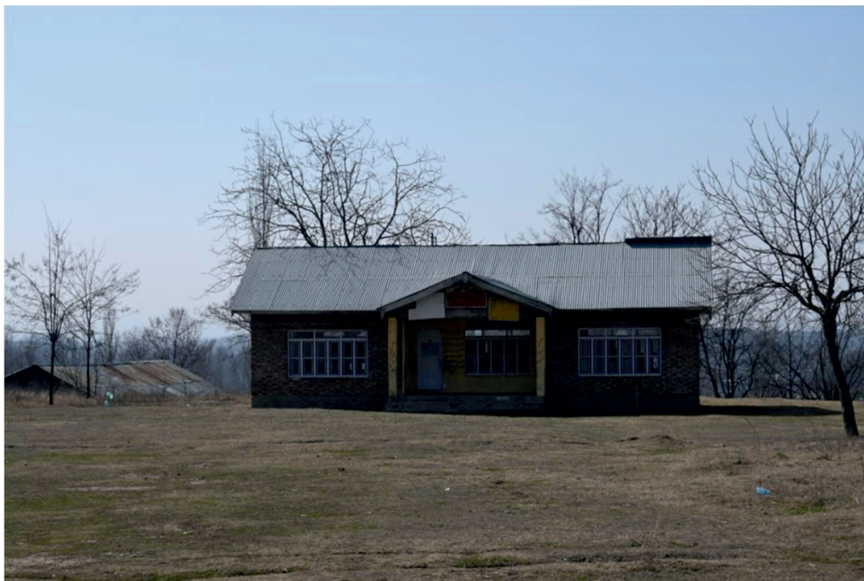
Figure 5: View of the School Building constructed on top of the archaeological mound (Image credit: Author)
