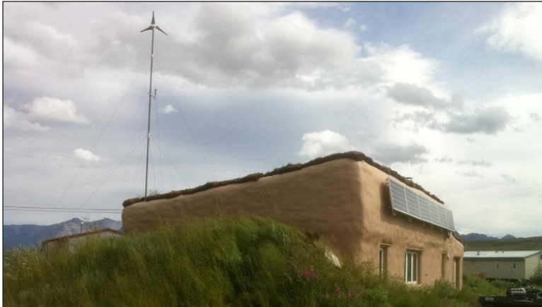
Figure 4 : The Anaktuvuk Pass Prototype Home, which incorporated traditional indigenous design with new sustainable systems. It was built in 2009 as a collaboration with the Tagiugmiullu Nunamiullu Housing Authority, village of Anaktuvuk Pass, Cold Climate Housing Research Center, and students from Iñisaġvik College. From the Cold Climate Housing Research Center: < http://cchrc.org/anaktuvuk-pass-prototype/ >.
